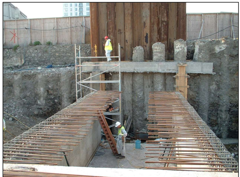
Figure 4.3 Tie-in of culvert to secant piled wall for future connection to Phase 2 culvert
